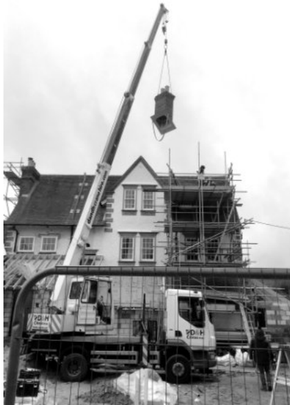
Installing the replacement chimney
