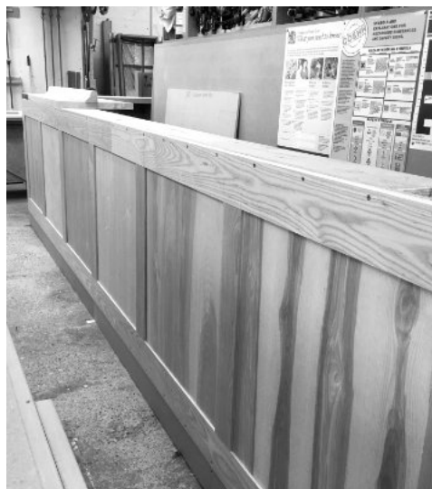
Sneak peek of the bar under construction.
